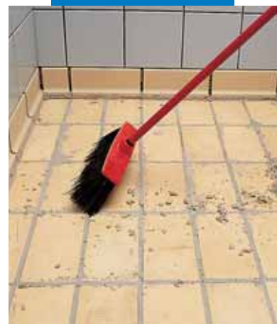
Removing the excess Kerapoxy SP with a broom
