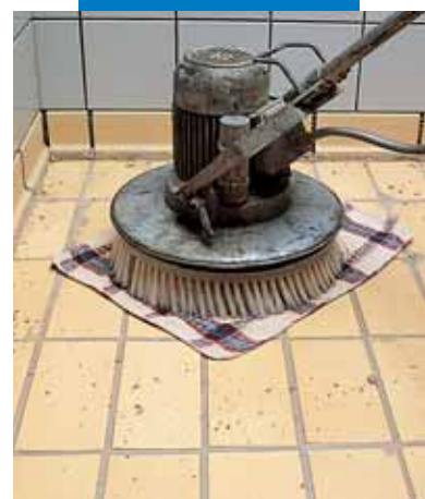
Cleaning with alcohol and a cloth using a rotary-disk type power float
